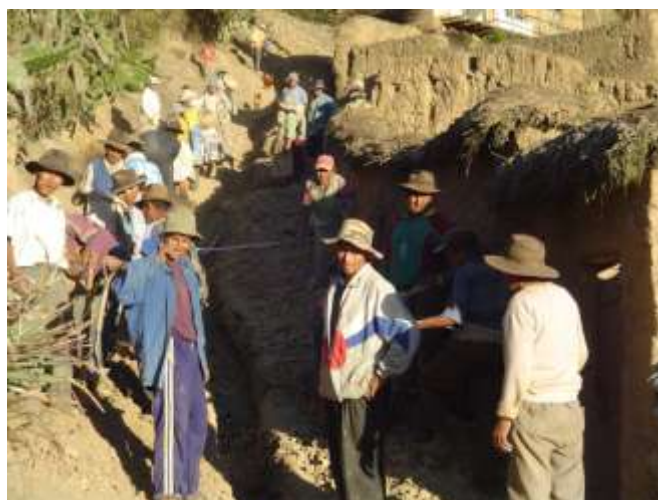
Community working to lay pipes
