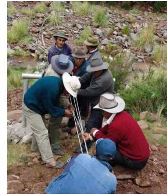
Men in Palcoma Baja working on their water project.
