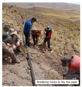
water from sources that are clean and protected from animal and soil pollution, and then providing an extended piped water system running within easy reach of all. The community themselves lay the many kilometres of pipe which often run over very difficult terrain.
